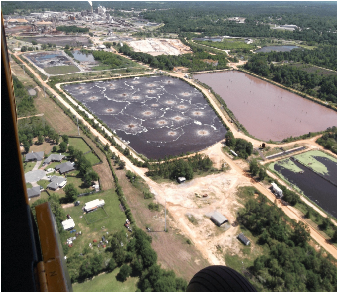
This is a picture of IP's large treatment pond called aeration stabilization basin.
